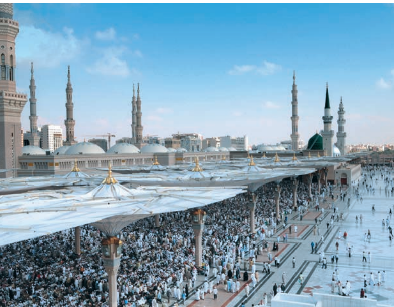
Aussenluftkühlung in Medina, Saudi-Arabien
